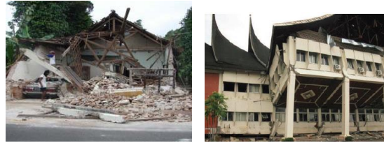
Damages due to Earthquake: Jogjakarta 2006 & Padang 2009
